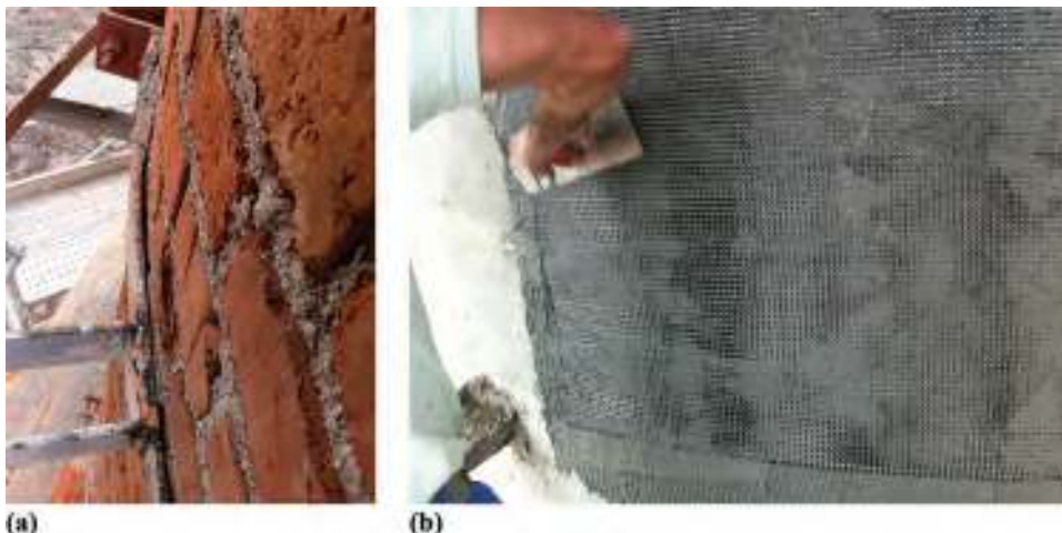
Fig. 4.2.1b—Chimney masonry surface: (a) before strengthening; and (b) during strengthening.
