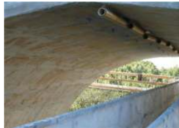
Fig. 4.1.2b—Details of work in progress (second fiber mesh).
