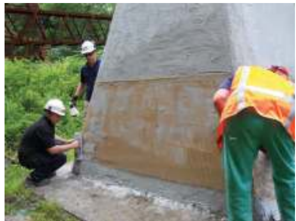
Fig. 4.1.4b—Installation of FRCM system.
