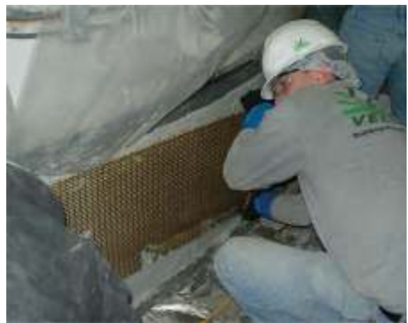
Fig. 4.1.5—Installation of reinforcement mesh on equipment base.
