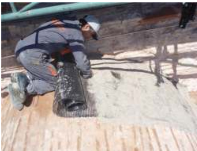
Fig. 4.2.3—Strengthening of clay brick masonry dome.
