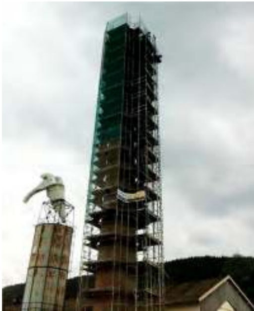
Fig. 4.2.1a—Chimney with scaffolding during repair.
